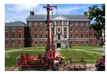
Rotosonic drill near historic hospital extracting continuous core down to 125ft.—through glacial till, original 19th century seawall, to bedrock.
