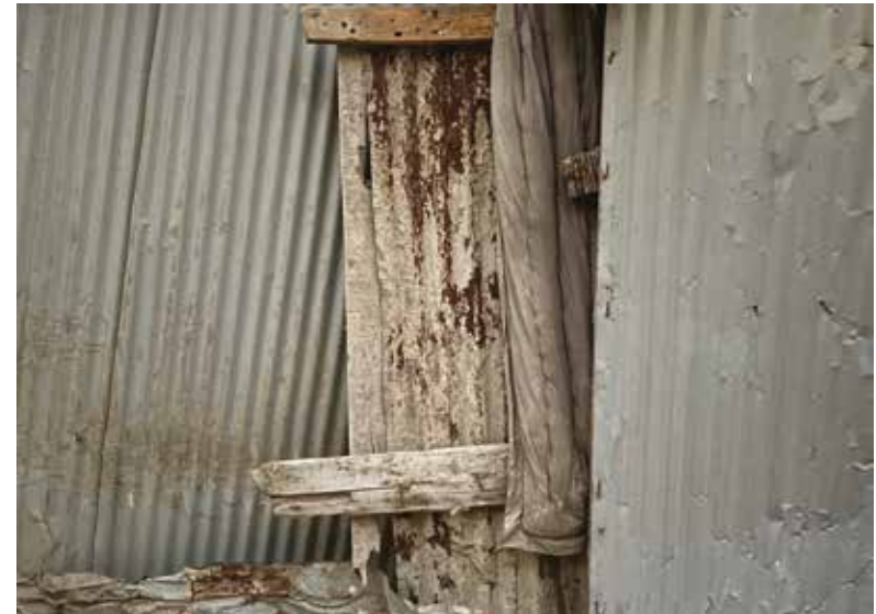
Space No.1 – Discarded corrugated metal sheets. Photo by author
